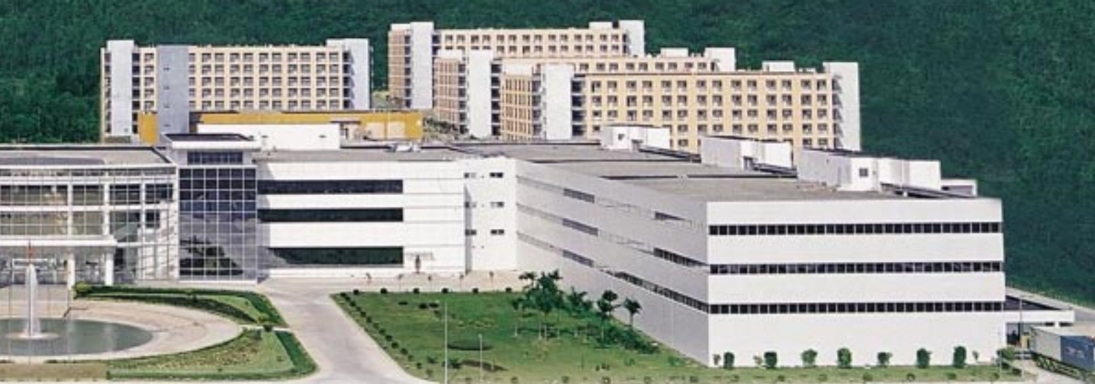
CCT Tech's Huiyang Manufacturing Complex
