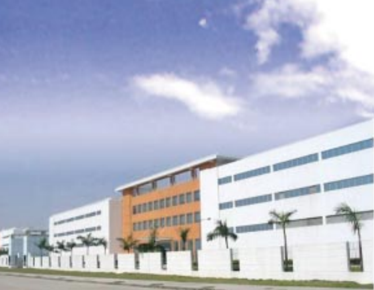
CCT Tech's Dongguan Manufacturing Complex
